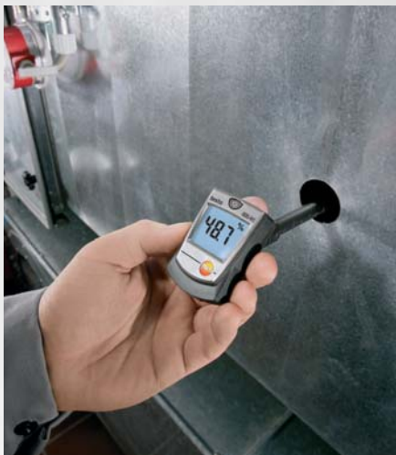
Monitoring air humidity in an air conditioning duct
