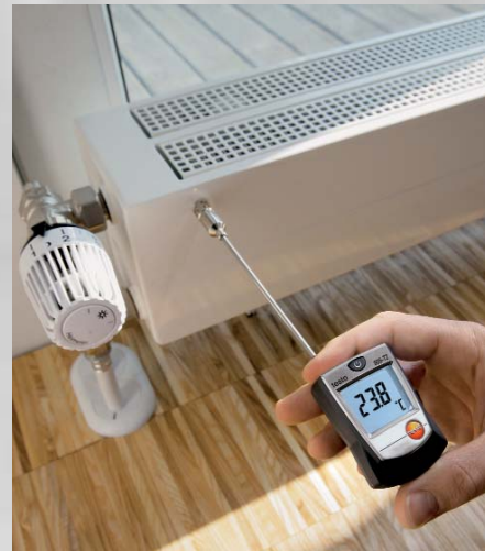
Surface temperature measurement on a radiator
